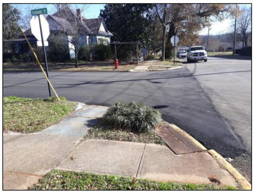
74 - Bloch St at Highland Two older style curb ramps need updating, lacking curb ramp in one direction
