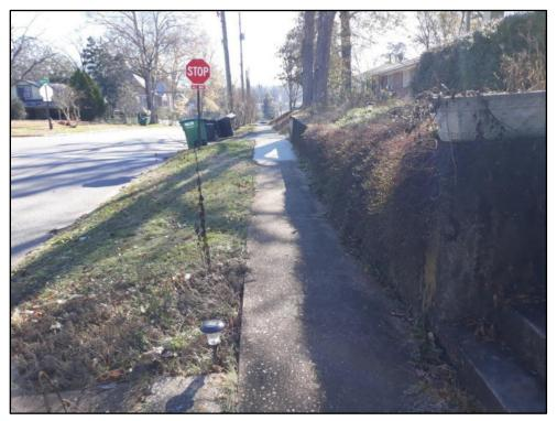
Shelby St between E Boundary and Alabama, south side Older sidewalk with some disjointed panels, width less than 48"
