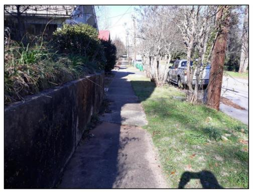
1 - Shelby St between E Boundary and Alabama Older sidewalk with some disjointed panels, width less than 48"
