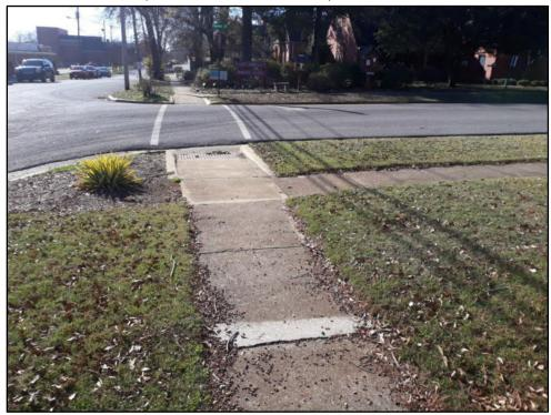
73 - Oak St at Plowman Updated curb ramps and sidewalk tie ins, also has had grinding to remove discontinuity
