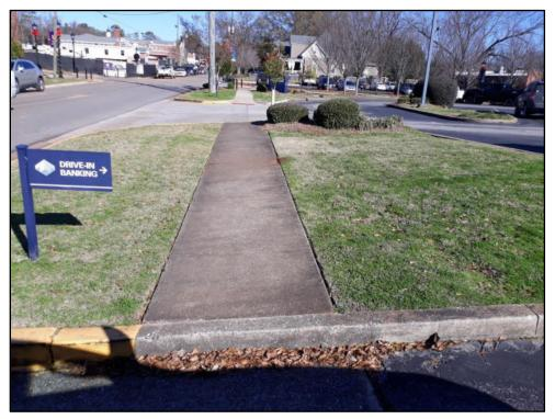
61 - Valley St from Vine to N Boundary Need 3 curb ramps installed on this block, 1 of which at alley currently has 2 steps
